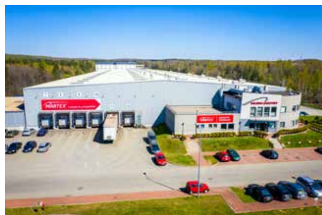
Central Warehouse - a bird's-eye view:
