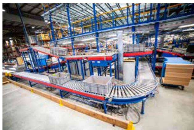
The new multi-level mezzanine
