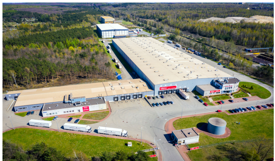
Central Warehouse, Dąbrowa Górnicza - a bird's-eye view
